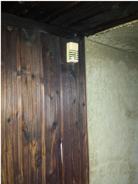
Internal lining Damaged and scorched
