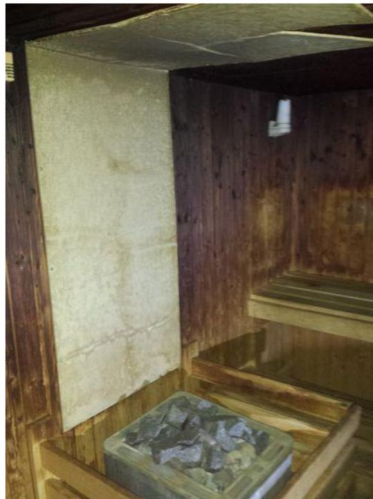
Heat proof lining Damaged Heater in poor condition.
